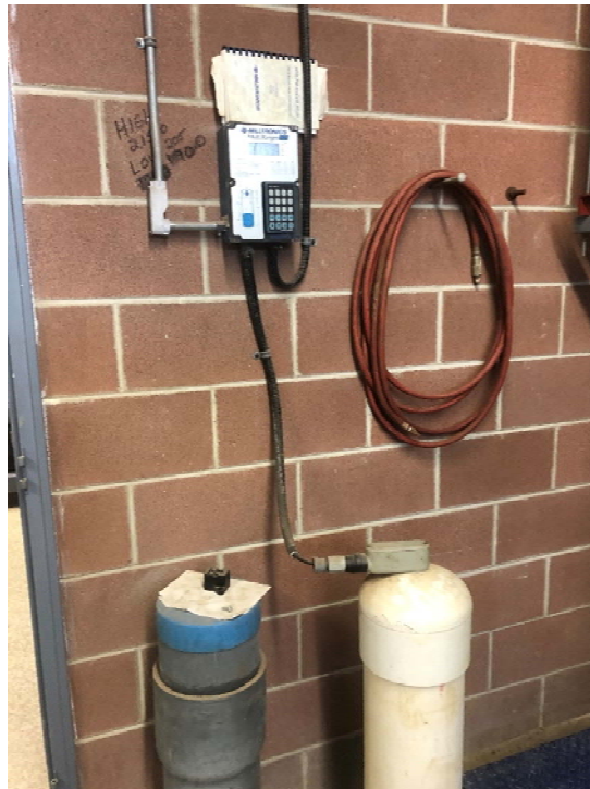
Water treatment plant reservoir level sensor
