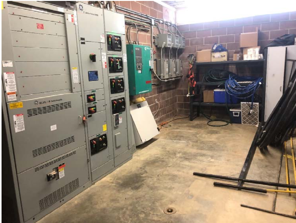
Electrical service equipment, motor control centres, and power transfer switch
