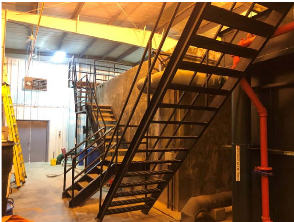
Flocculation chambers (center) and filters (right)
