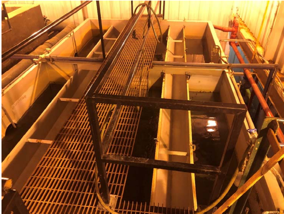
Filter compartments and access platform
