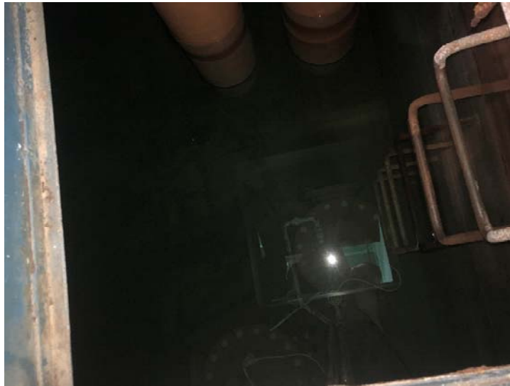
Pump well and flow control valve (sub-surface)
