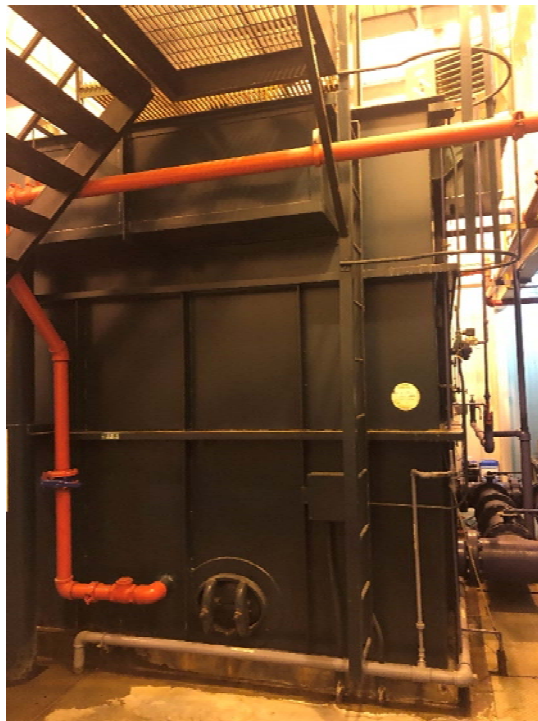
Mixed media gravity filters
