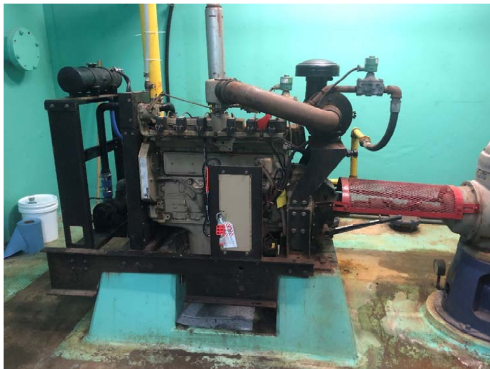
Standby motor and right angle-drive turbine pump
