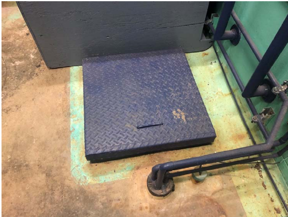
Pump well access hatch
