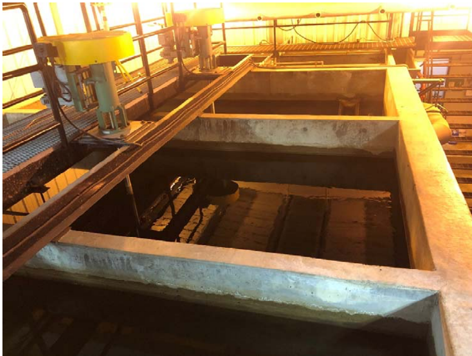
Flocculation chambers and paddle wheel motor (left)
