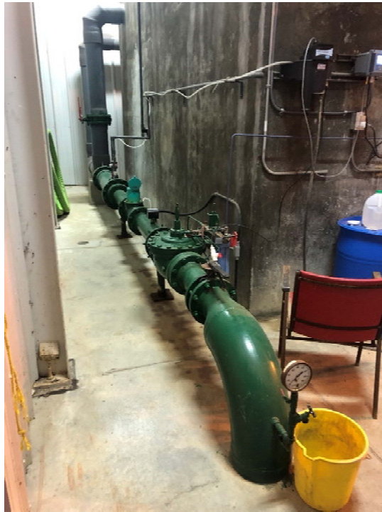
Raw water header piping and instrumentation
