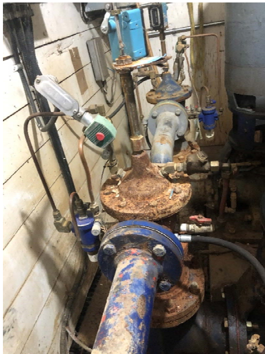
Raw water header piping and control valves
