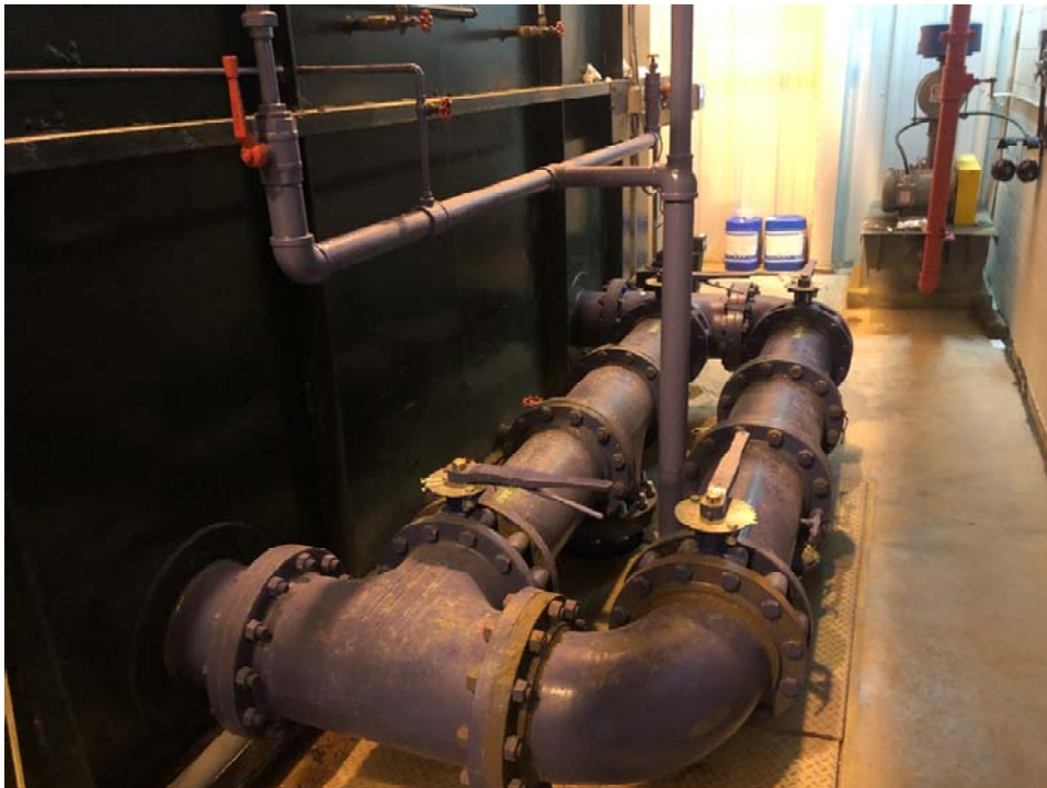
Filter effluent and backwash feed piping
