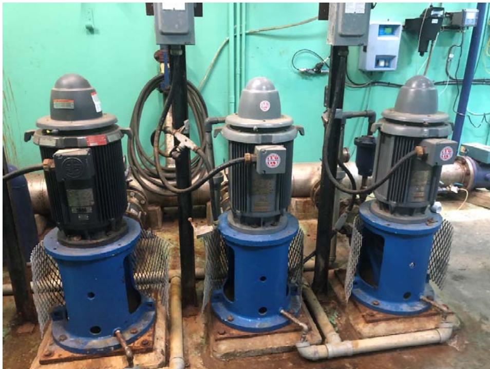
Vertical turbine distribution pumps
